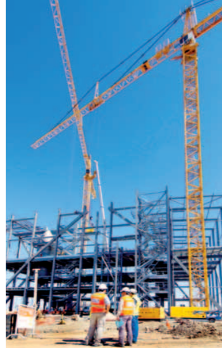
▲ Work is progressing well on the ANDRITZ recovery boiler.
