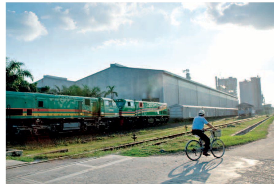
▲ The PT TEL mill has become part of daily life in South Sumatra, providing jobs and well-being for many people in the area.
