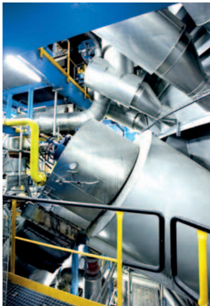
▲ The PowerFluid HC boiler has four feed lines to proportion fuels based on market price and availability. Natural gas is only used for start-up via the burners shown here. Emissions are well within targets.
