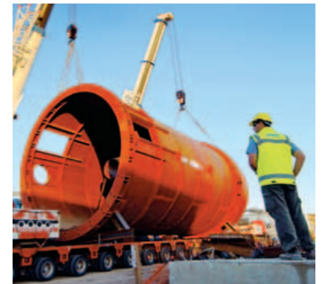
▲ Above: Preparing the foundation for a bleaching tower (fiberline building in background).
