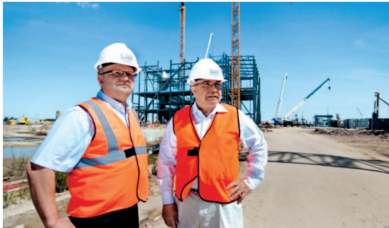
▲ With the ANDRITZ recovery boiler taking shape behind them, Eloranta of Stora Enso and Vivanco of Arauco represent the owners on-site. They offer executive support to the project and mill teams. “We started out as colleagues, but have become friends,” they say.
