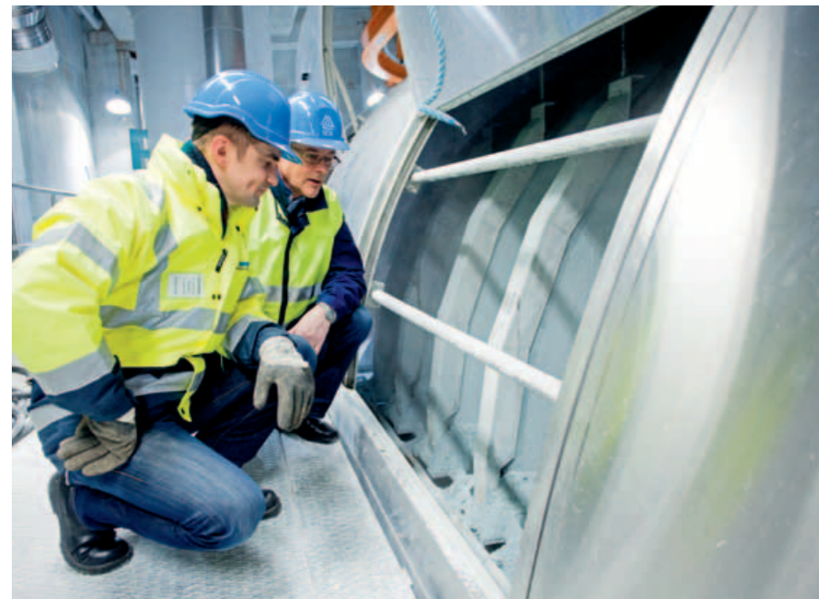
▲ A view of the LimeDry filter for drying lime mud prior to burning in the kiln. ANDRITZ also delivered a LimeWhite filter to enable the mill to meet future targets for white liquor production.
