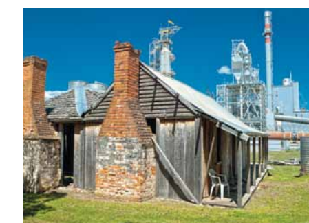
▲ Visy has restored local pioneer homes on the property with great respect to the original structures.
