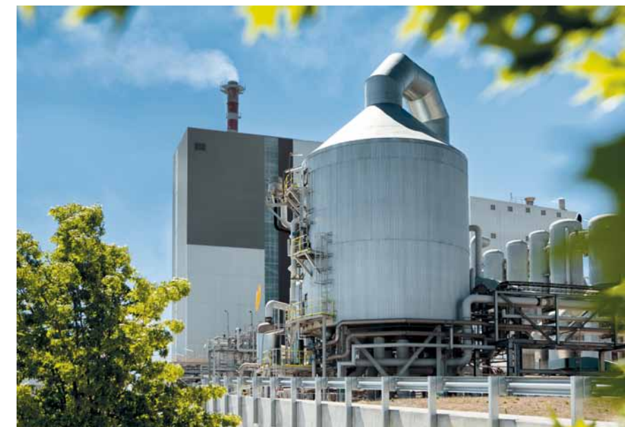
▲ Visy is home to the world's largest pulp mill VCE evaporator, delivered by ANDRITZ (in foreground). It is central to the mill's ability to minimize fresh water usage. In the background is the new ANDRITZ recovery boiler, expandable to 1,100 tds/d, which plays an important role in eliminating mill odors.
