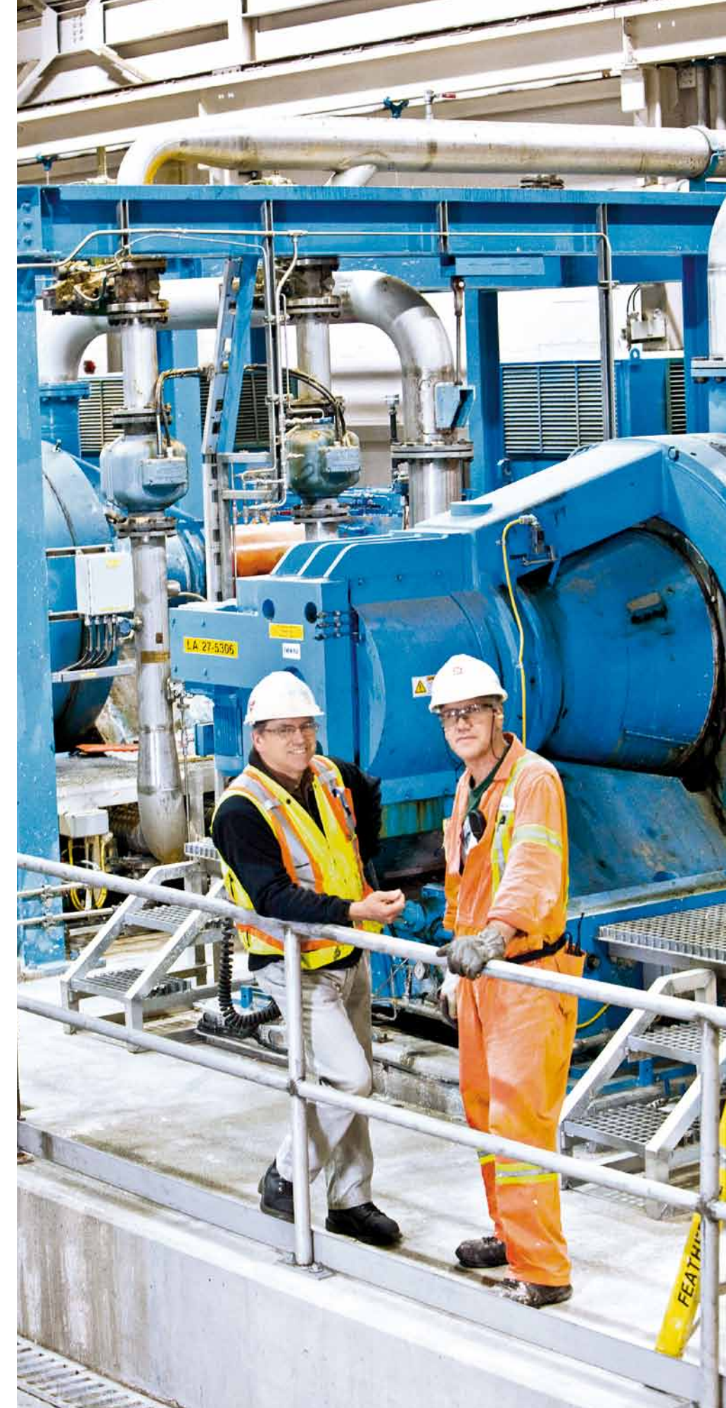
▲ The Crofton mill has three TMP lines equipped with ANDRITZ refiners. Production now approaches 900 adt/d.
