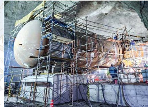
Beginning of 2023, the pressure test for the bifurcator of Asahan 3 was successfully executed.
