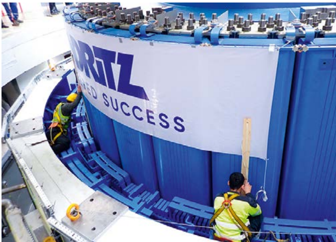
Installation of the generator rotor into the pit of Unit A-1
