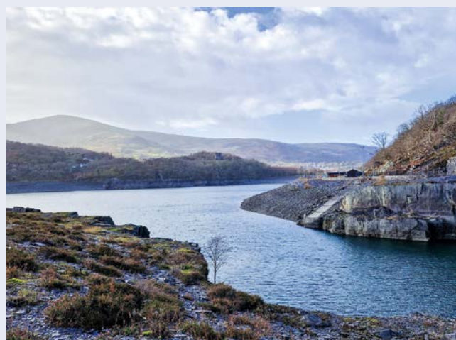
With a total capacity of 1,728 MW, Dinorwig is one of the largest pumped storage power plants in Europe.
