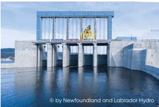
Intake gates including trash racks
