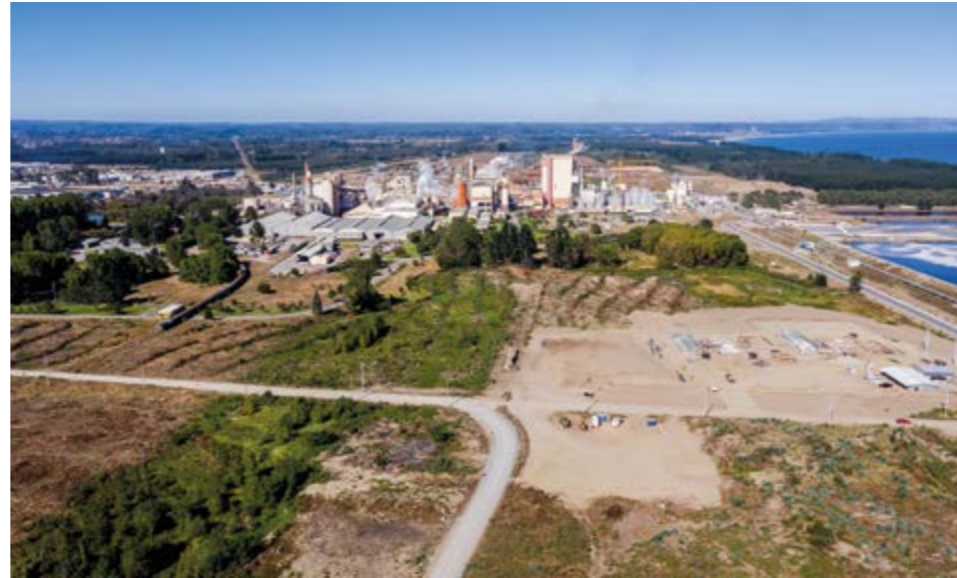
Arauco is planning to close the existing eucalyptus line L1, upgrade the existing pine line L2 and install a new state-of-the-art eucalyptus line L3.
