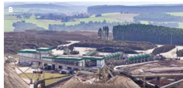
A The white liquor plant delivered by ANDRITZ in 2016 for Klabin's pulp mill in Ortigueira, Paraná, Brazil, has one of the world's largest recausticizing plants, with 16,000 m 3 white liquor production daily.
