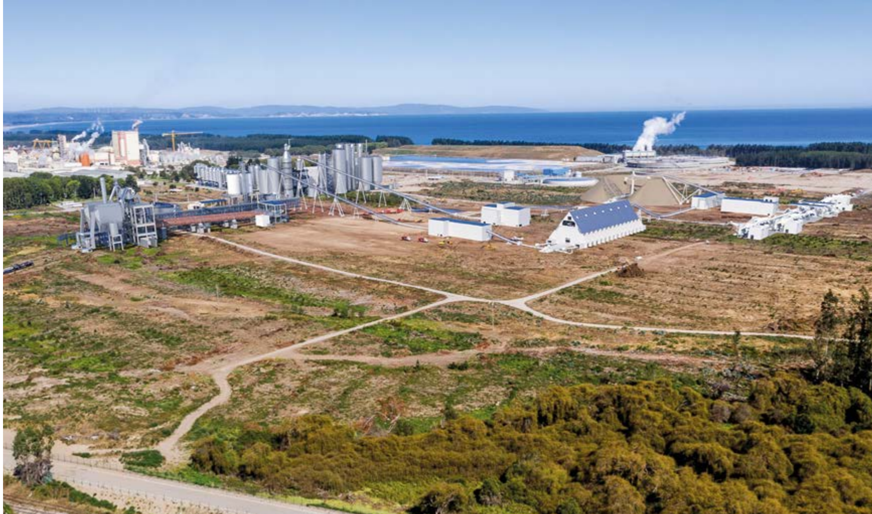
After start-up in 2021, Arauco's Mill in Horcones will be the most modern mill operating in the 21st century.
