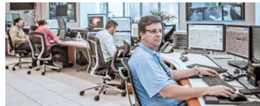
The control room at Eldorado is the action center for production control. OPP software resides in the DCS for advanced control of fiberline processes and also links process, maintenance, and asset management information into one network.
