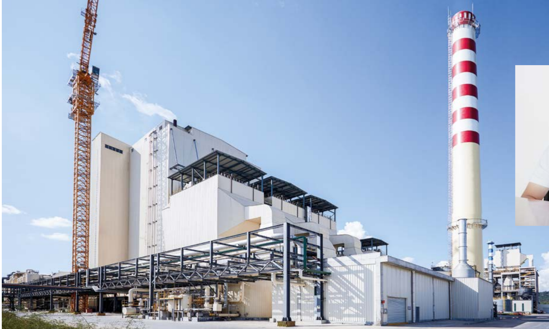
ANDRITZ supplied the mill with the largest HERB recovery boiler in Laos with a capacity of 2,200 tds/d, in order to secure safe and reliable operation.
